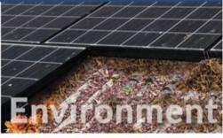
Leaves and Debris collect causing rot and fire hazard
